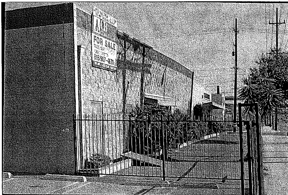
Figure 13 – The masonry wall at the right front of this building has pulled away from the roof. This can be a serious problem in buildings with concrete block or tilt-up concrete walls that have wood roofs.
