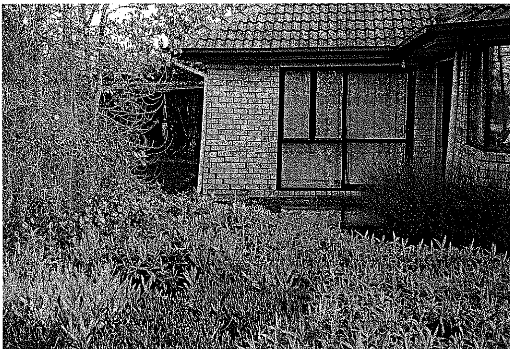
Figure 10 – Example of liquefaction damage to a house after the magnitude 6.3 February 22, 2011 Christchurch, New Zealand earthquake. The house was undamaged by shaking but seriously damaged by ground movements caused by liquefaction.
